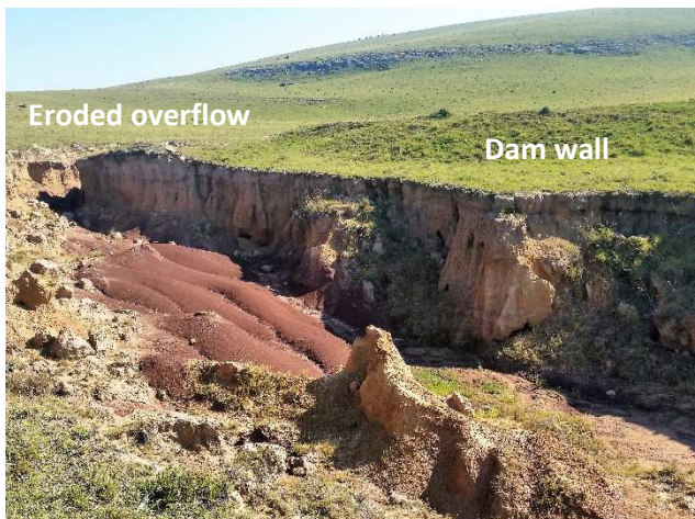
Plate 5. Eroded dam wall upstream of proposed water release point, looking upstream.
