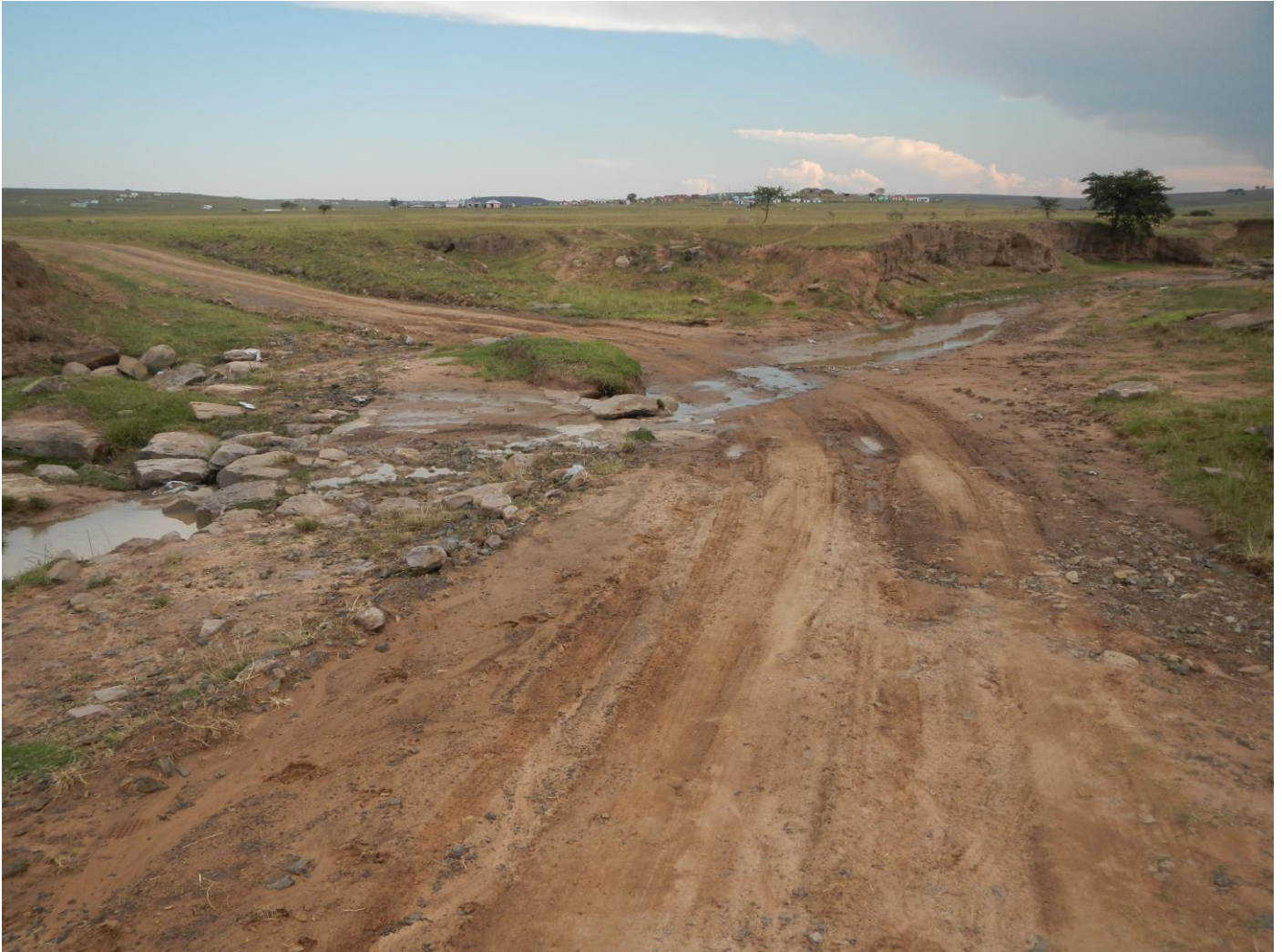
Figure 11: Image of the main drift crossing the Toboyi River.
