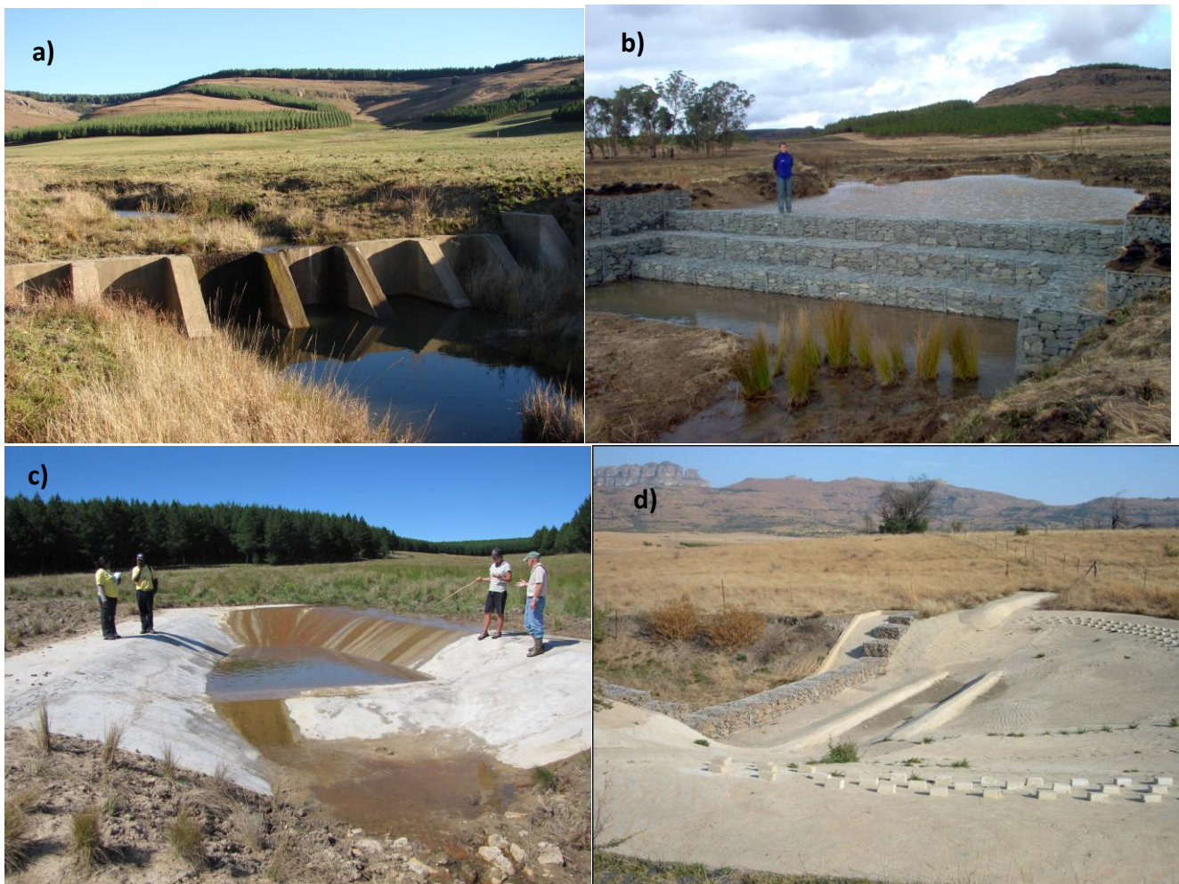
Figure 9: Examples of headcut control structures: a) weir, b) gabion, c) and d) chute (photos by J Buckle).
